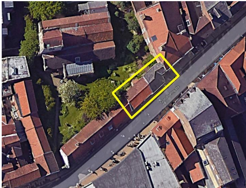
Figure 2. Aerial view of 60 Goodramgate with the tile (left) and slate (right) roofing systems.
