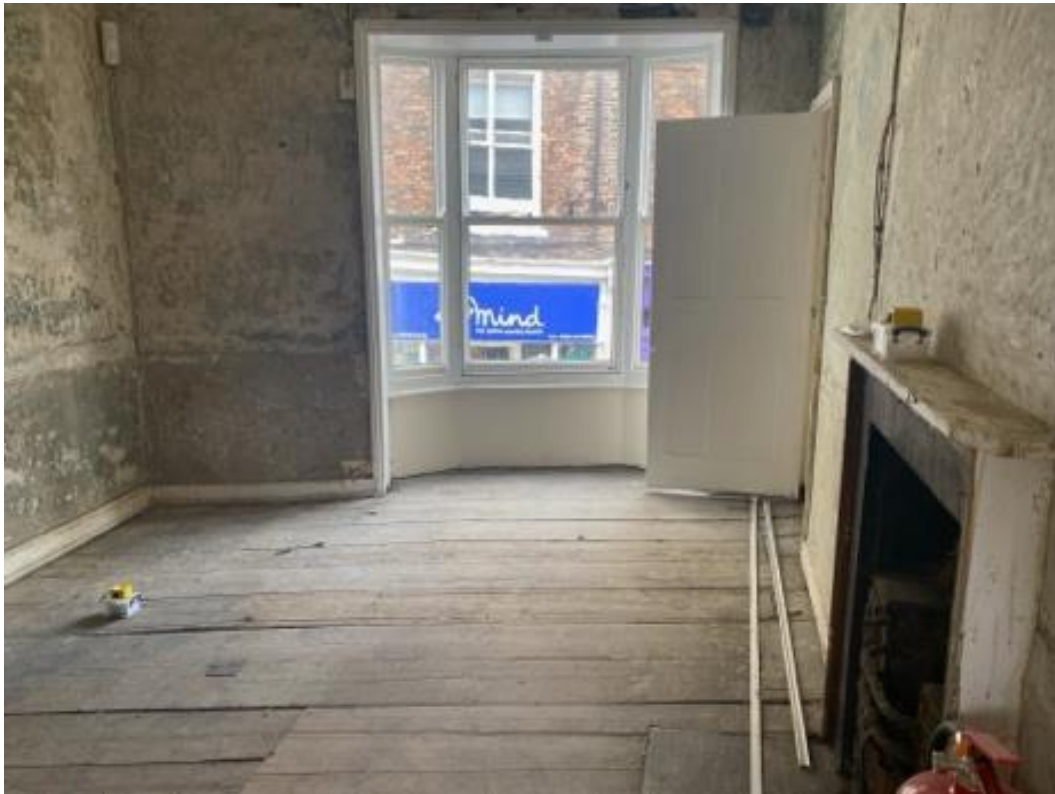
Figure 4. Location of logger BLF1 (left) and logger BLF2 (right).
