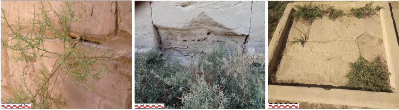
Figure 2. Shows growing higher plants in different area of the temple causes some deterioration features
