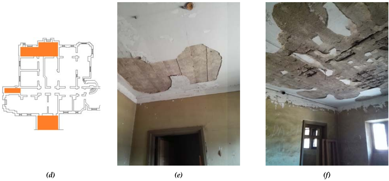
Figure 7. Falling down of the concrete cover of ceilings: (a) first floor ceiling damaged parts, (b) and (c) samples from damage, (d) basement floor ceiling damaged parts, (e) and (f) samples from damage.
