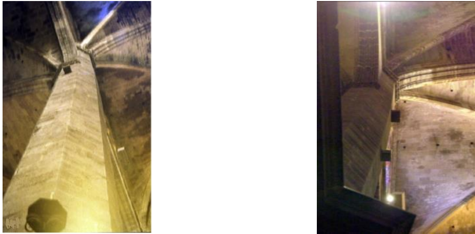
Figure 10. Deformed columns: internal column (left); and column at triumphal arch (right).
