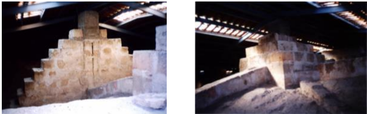
Figure 7. Additional weights: over the transversal arches keys (left); and over the vaults keys (right).
