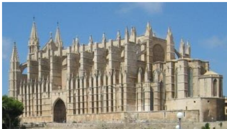
Figure 2. Mallorca Cathedral: external view showing the apse area and the south façade.
