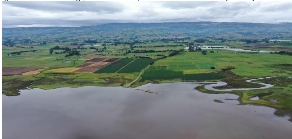
Overflow Of the Copa Dam- 2023. Photo: Dora Marcela Benítez Ramirez.
