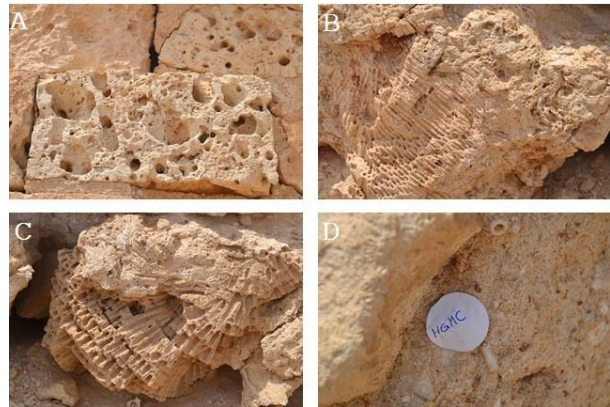
Figures 52. Four different shots from Farasan islands (German house) showing the effect of wind on building stones (A), the typical shape of coral building limestone (B,C) and the high amount of shells and fossils in plaster layer (D)
