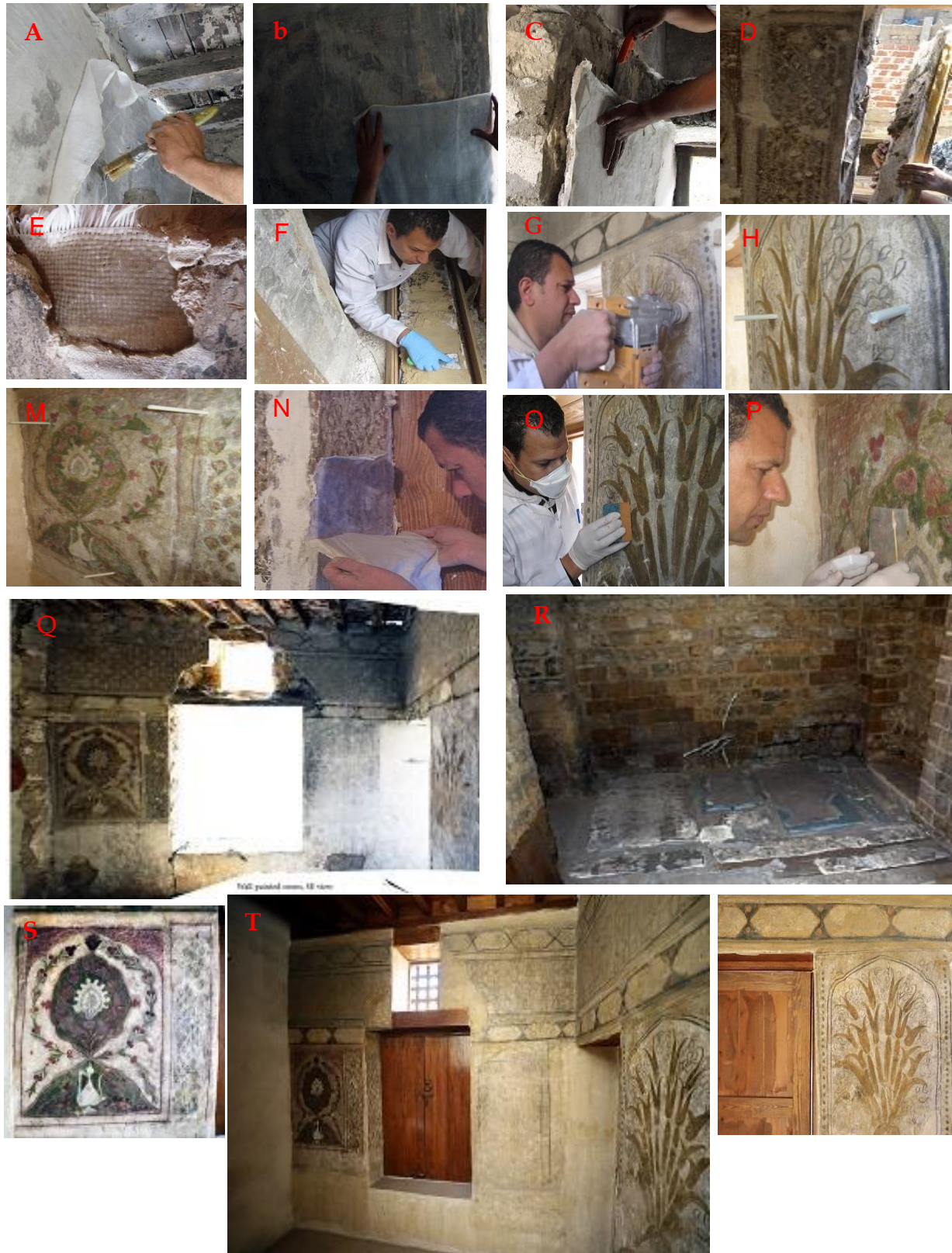
Figure 11. Treatment, restoration detachment and re-attachment steps (a, b); Apply a surface protection layer (facing) Before detachment (c); the tools used for sawing. mural painting after detachment (d); During detachment (e, f); Add a fiberglass layer to strengthen the mortar (g,h,m); During re attachment the murals painting with the fiberglass bars (n); Remove the facing layer (o, p); cleaning the colours by wash up and chemical cleaning (s); mural painting before detachment (r); Wall paintings after detachment (s, t, u); Wall paintings after re-attachments) mural painting before detachment (r); Wall paintings after detachment (s, t, u); Wall paintings after re-attachment.
