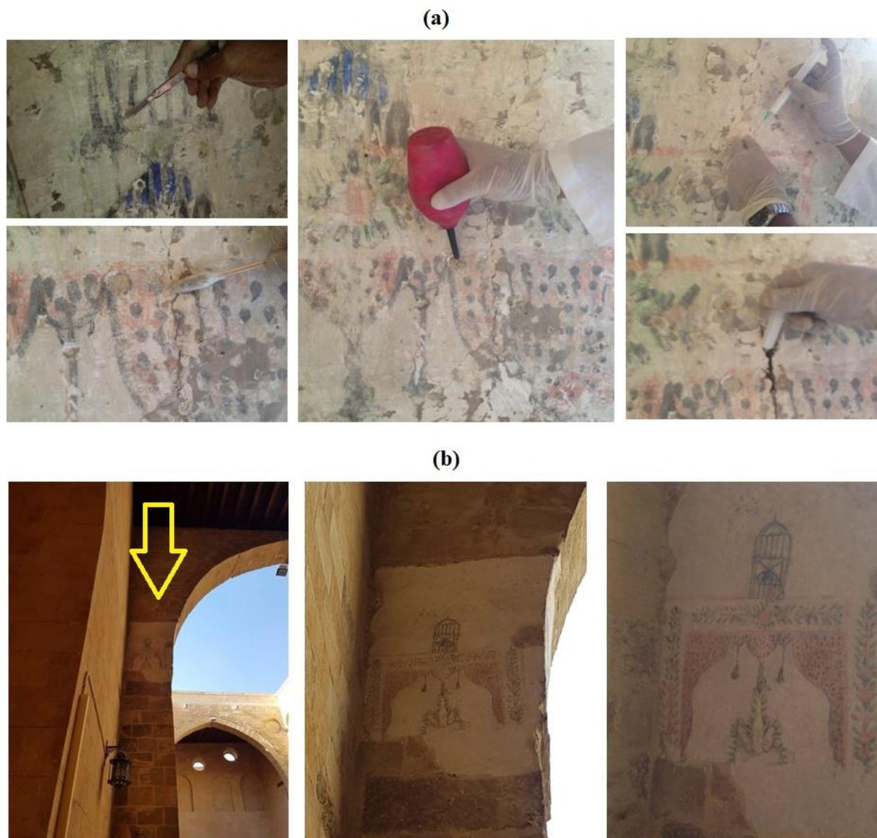
Figure 13. a) examples of the restoration procedures applied to the murals (e.g. cleaning, injection of open cracks, etc), b) the studied mural after the final steps of restoration (the yellow arrow refers to location of the mural).
