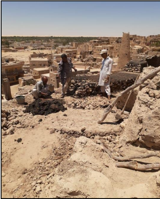
Figure 9. The people used the same old construction technique with Al-Kurshef in building modern houses
