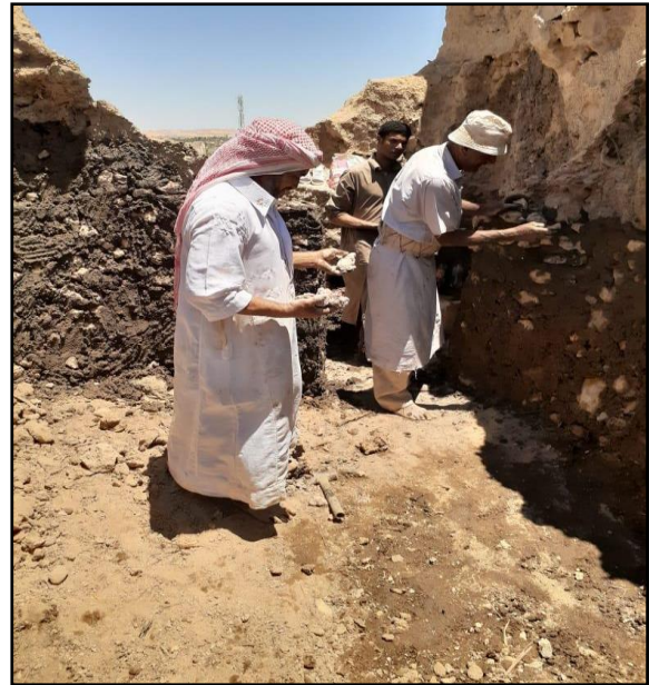
Figure 10. Building a modern wall using Al-Kurshef
