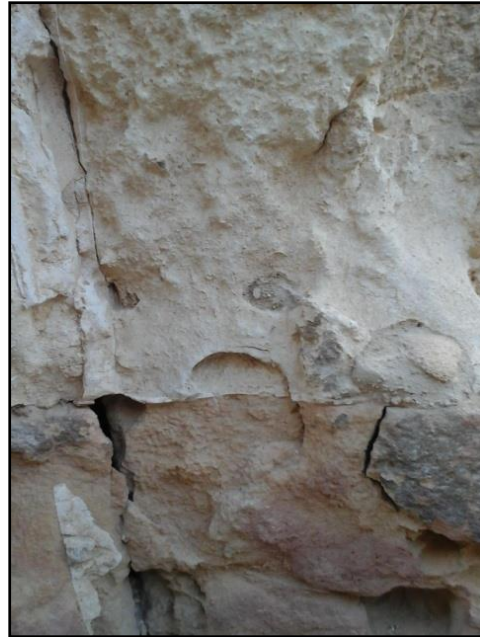
Figure 23. the crumbling of the saline limestone surface as a result of the saline geological nature of the Siwa Oasis - the Oracle Temple
