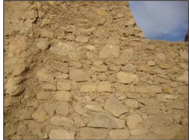
Figure 6. Building with Al-Kurshef blocks and mortar in the historic Shali Castle
