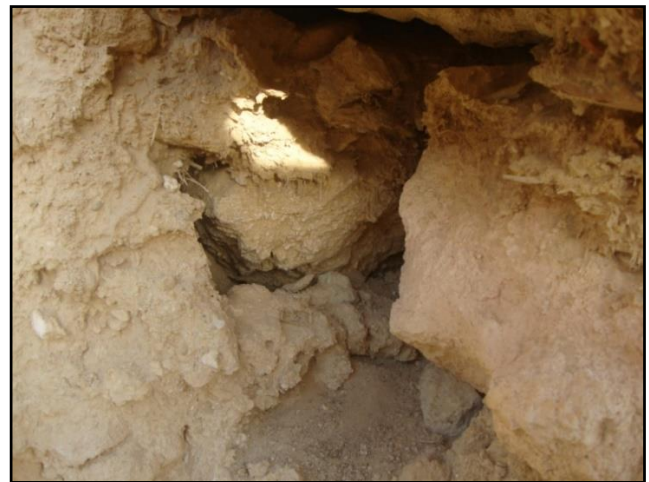
Figure 29. The weakness and fragmentation of Al- Kurshef in the eroded part of the walls - the historic Shali castle
