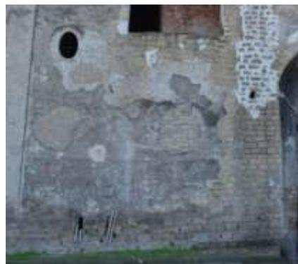
*Figure 4. Crushing phenomena on masonry walls*
