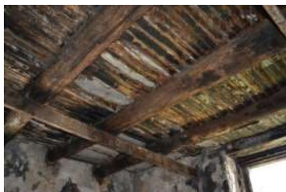
*Figure 7. Widespread phenomena on the wooden floor - The fall of the planking*
