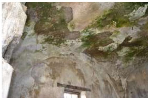
*Figure 3. Injuries on the intrados of masonry vaults*
