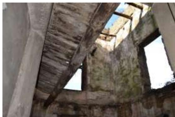
*Figure 5. Widespread phenomena on the wooden floor - Partial collapse*
