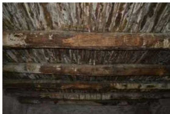
*Figure 6. Widespread phenomena on the wooden floor - Inflection on the main beam*
