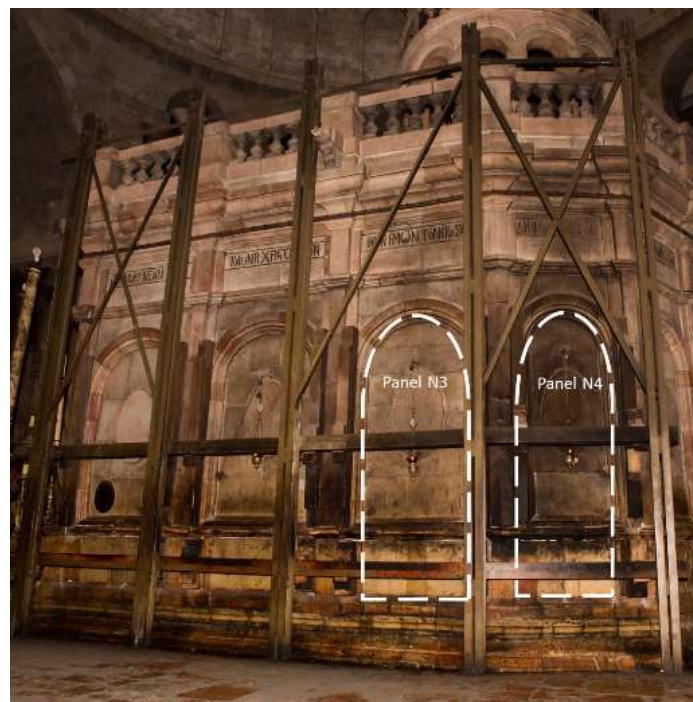
Figure 5. The North side of the Holy Aedicule before the rehabilitation works. In the white frames the two panels where the GPR measurements took place (photo courtesy of A. Moropoulou)
