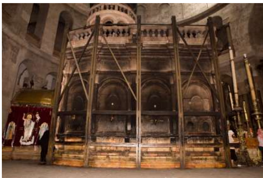
Figure 1. The south side of the Holy Aedicule prior to the rehabilitation works (photo courtesy of A. Moropoulou)
