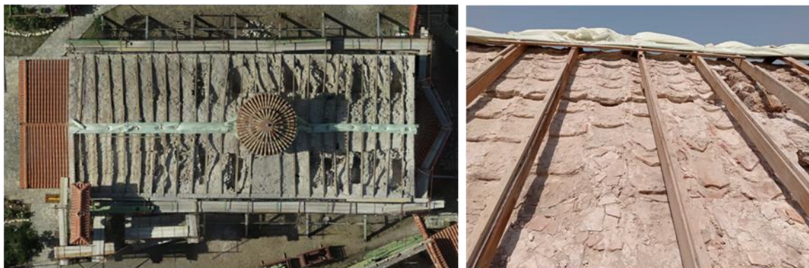
Figure 4: Revealed roof construction (left: orthomosaic, right: detail of construction)
