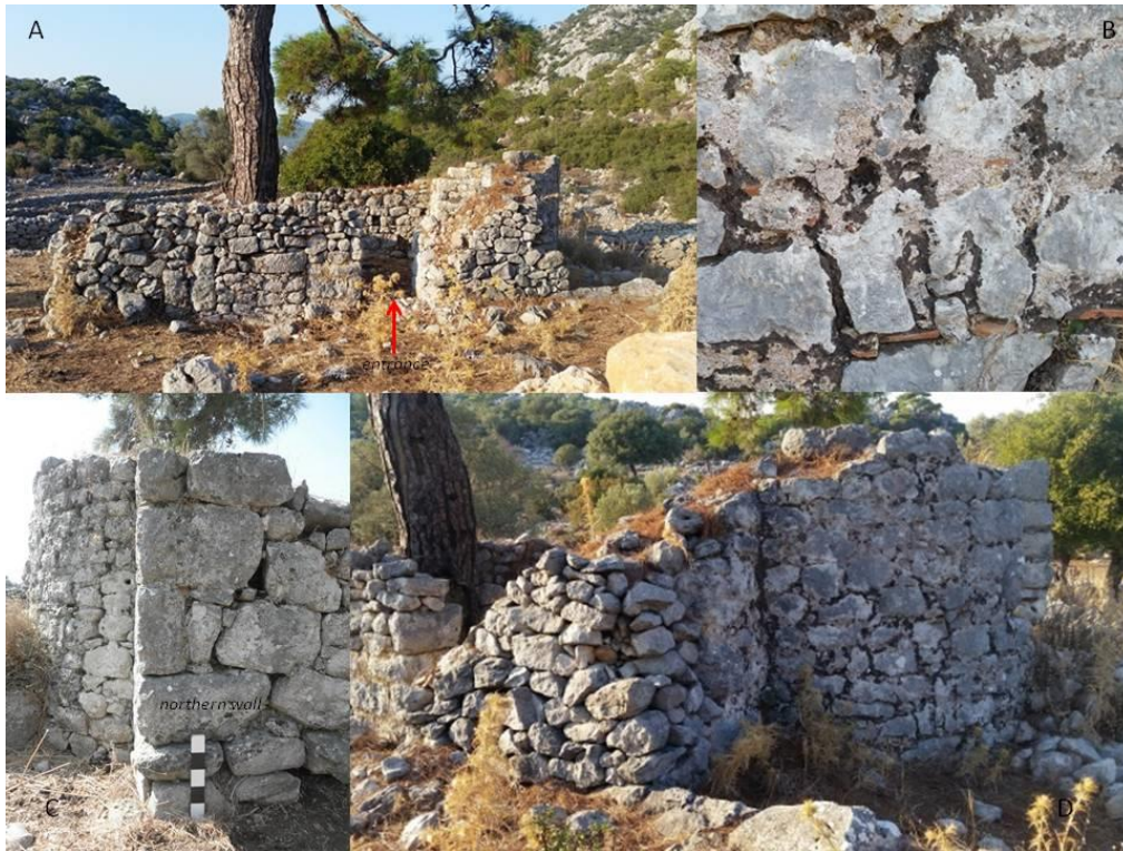
Figure 12. Close-Up Position of the Church (A); Detail of Masonry (B); View From the Corner of Northern Wall (C); View From Opus Incertum (D) (Photographs by Author)
