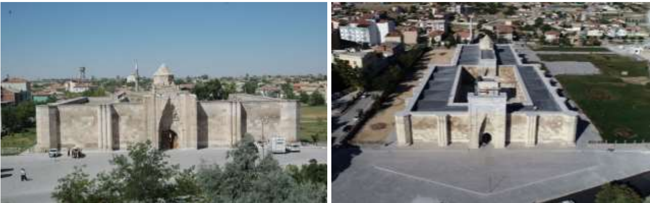
Figure 18. Sultan Han, before (Url-13) and after (Url-14) restoration.
